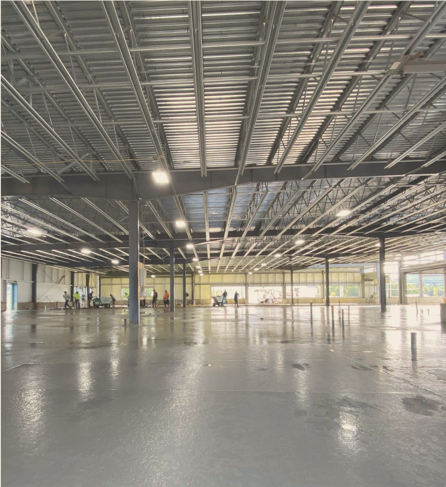
River Valley Co-op, Easthampton, MA under construction
